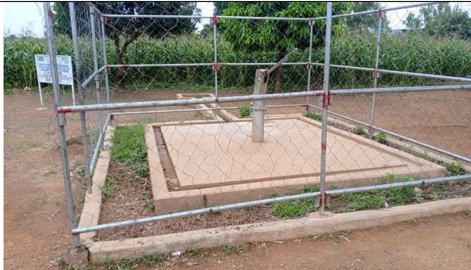
Photos of the village's only hand-driven pump, installed in Tabota's A-B public school.
