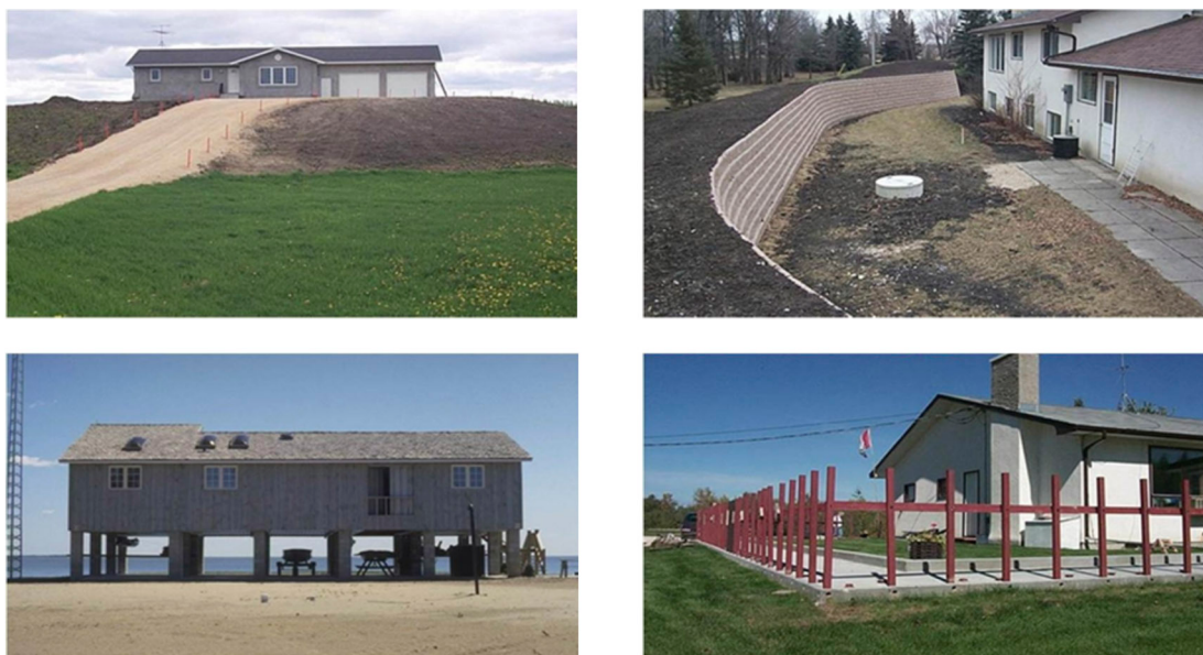
Figure 13 — Other methods of floodproofing: raising (top and bottom left); retaining wall (top right); removable structural dyke (bottom right) (Paul Pilon)
