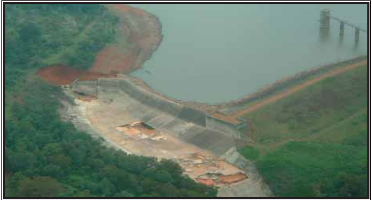
Figure 10: Damage to Sasumua Dam July 2003
