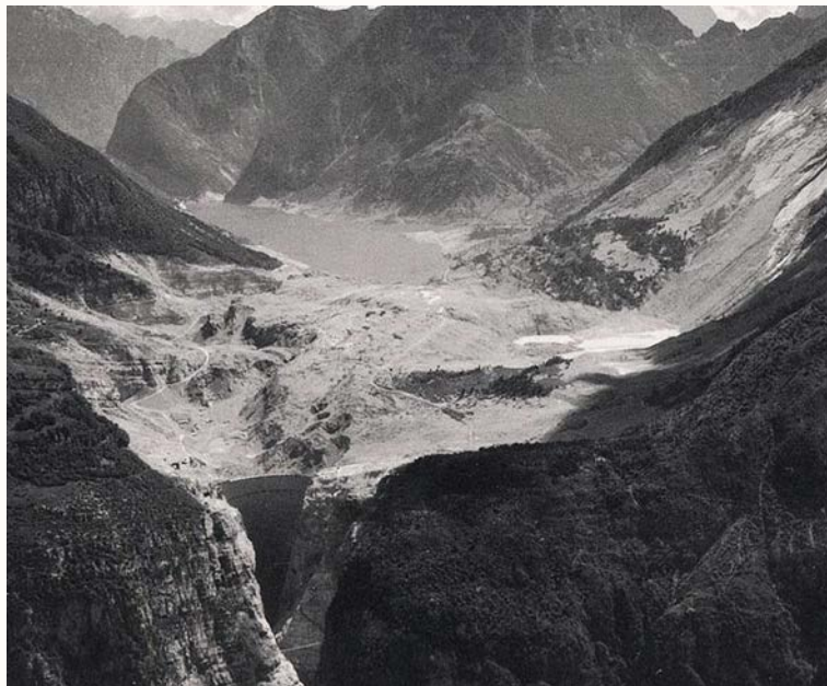
Figure 7 — The Vajont Dam after the landslide occurred in October 1963 (CFBR, 2012)
