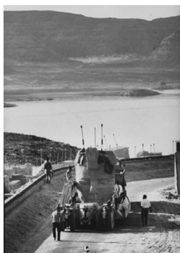
Figure 13 — Sandstone head of Ramses II being moved to be reassembled at the new site of Abu Simbel, 1966, in view of submersion of the original site due to the construction of the Aswan High Dam. (Photo: © Terrence Spencer/Time and Life Pictures/Getty Image)
