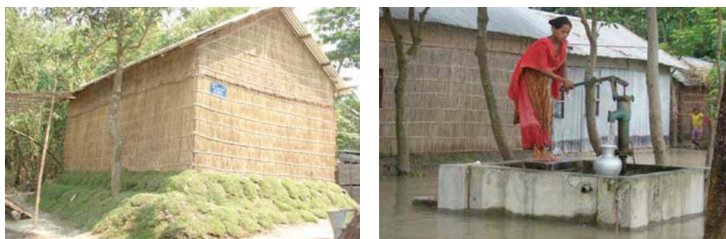
Figure 7 — Raised house and tube-well enable families to cope with floods (Practical Action Bangladesh, 2010)
