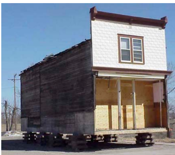
Figure 12 — Relocation of the Boomtown Building after the 1997 Red River flood in Grand Forks, North Dakota (FEMA, 2001)
