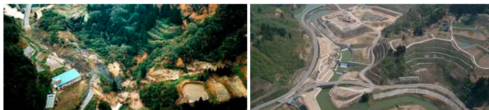
Chuetsu Earthquake; 2004, Niigata Pref., Japan (Left: Just after occurrence, Right: Countermeasures completed)
