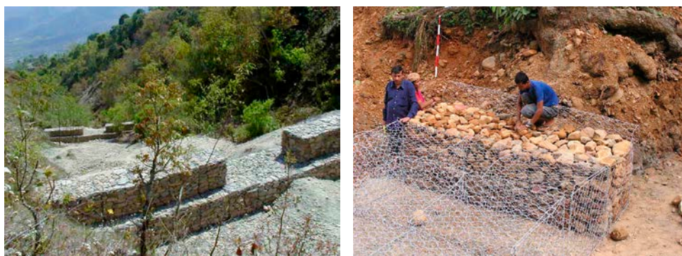
Series of Gabion sabo dams; Dahachowk, Nepal
