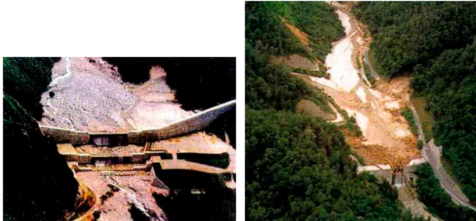
Sabo dam No. 1 on the Name River in the Nagano prefecture, Japan
