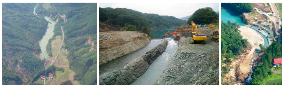
The Iwate-Miyagi Inland Earthquake; 2008, Iwate and Miyagi Pref., Japan (Construction of an emergent drainage channel to lower water level; Just after earthquake; Countermeasures completed)
