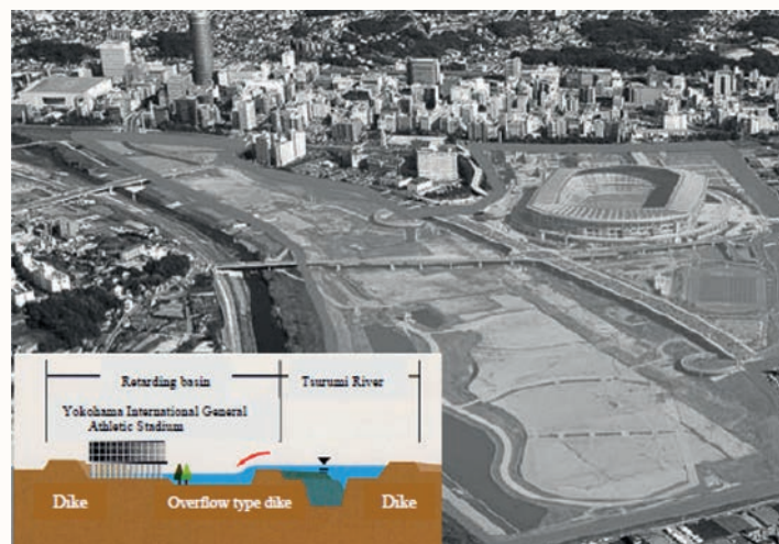
Figure 35 — Tsurumi multi-purpose retention basin (Jha et al., 2012)
