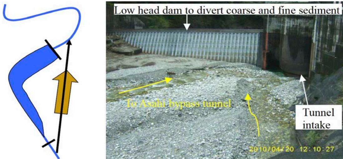
Figure 12 — Coarse sediment load bypass around an Asahi in-stream reservoir using a bypass tunnel (Sumi and Kantoush, 2010)
