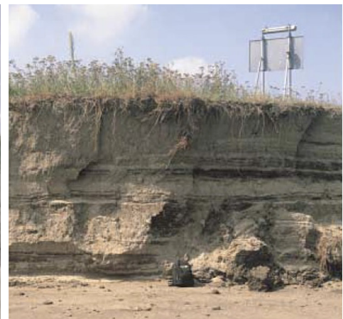
Bank erosion near the intake of one of the secondary channels (photo L. Jans).
