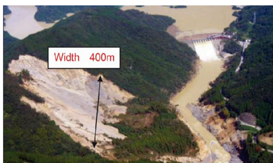
(a) Slope failure downstream of the Tsukabaru dam
