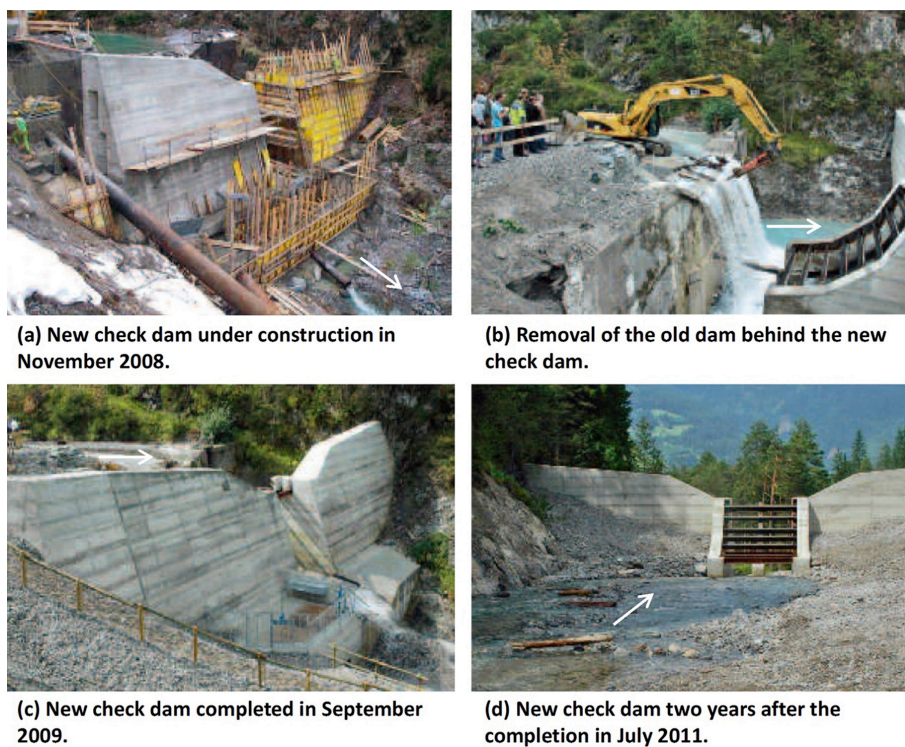
Figure 27 — Construction process of the open check dam at Feistritzbach (Carinthian state government, 2011)
