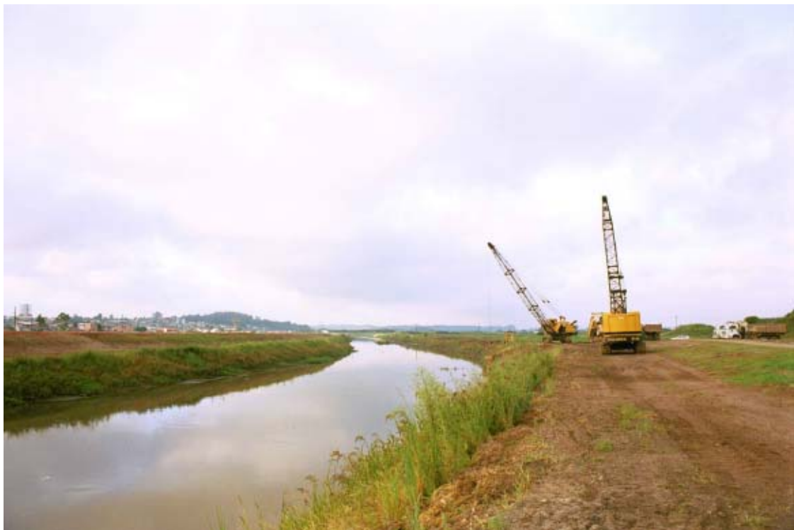
Figure 8 Channel under construction (parallel to Iguaçu River)
