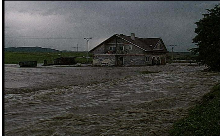
Photo 4. The flood situation on Štrbský Creek in Štrba village
