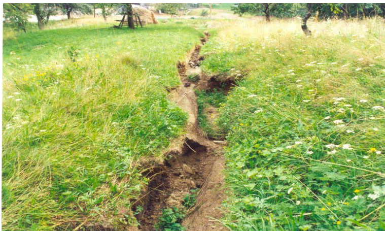
Photo 8: The erosive gouge on the left slope of Malá Svinka valley (the depth 1,5 m) in the village Uzovské Peklany
