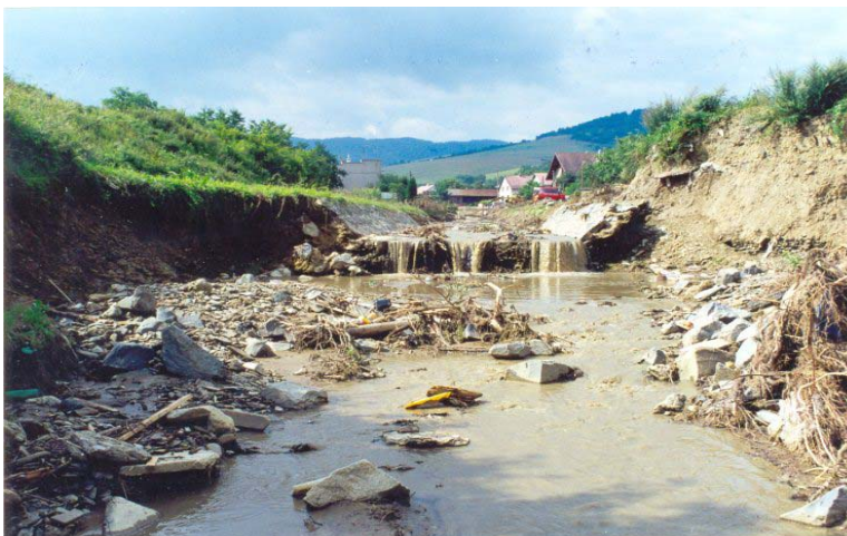
Photo 1: Dubovický creek - The end of stream regulation destroyed by back erosion
