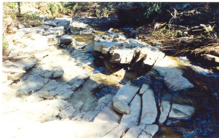
Photo 4: Eroded channel of Malá Svinka down to bed rock (cracked desks of sandstones)
