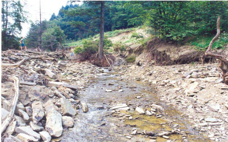
Photo 5: Eroded channel of Malá Svinka (landslide of slope from 5 to 8 m), the creek channel silt up with branches and stones and rocks)
