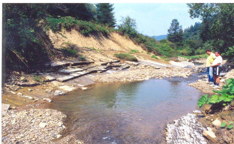
Photo 10: Eroded left bank of the creek channel (down to bedrock) of Renčíšovský creek above the village Renčíšov
