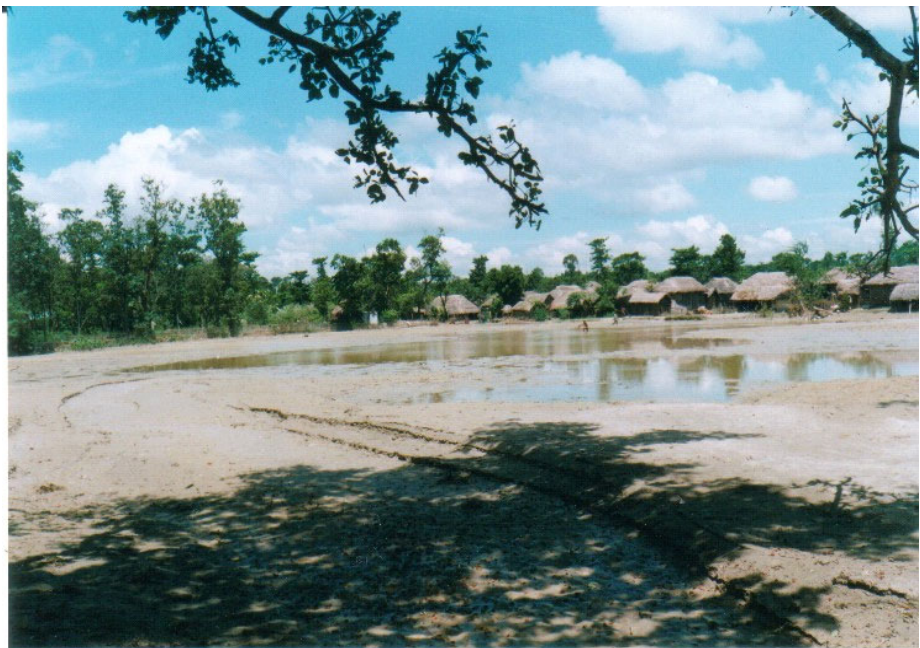
Fish pond silted up by sediment deposition
