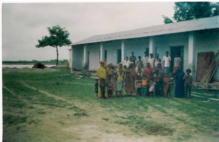
Bramhapuri VDC Lower secondary school on Bagmati river bank. It was swept away on 31st July, 2003 Flood.
