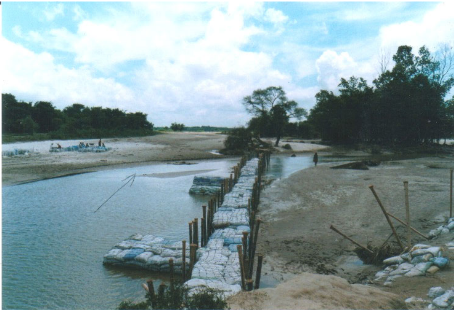
Reconstructed embankment made of bamboo pile, sand bags in gabion boxes
